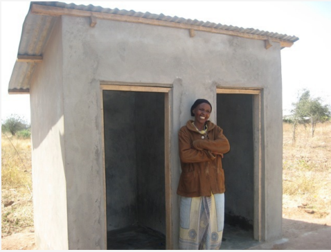
Safe toilet constructed by Dismas and his family.
