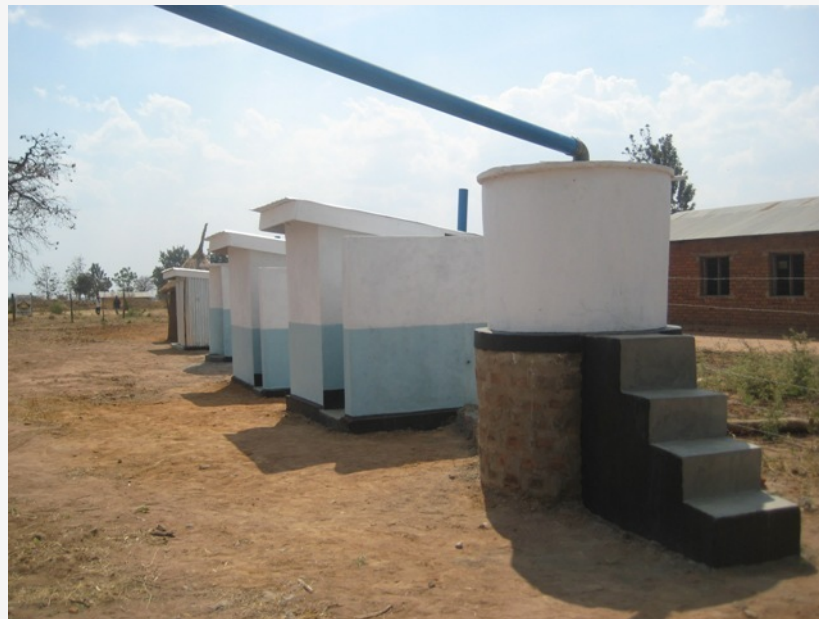
The image shows the several toilet options with different technology and cost for the community to learn and uptake the technology to their homes.
